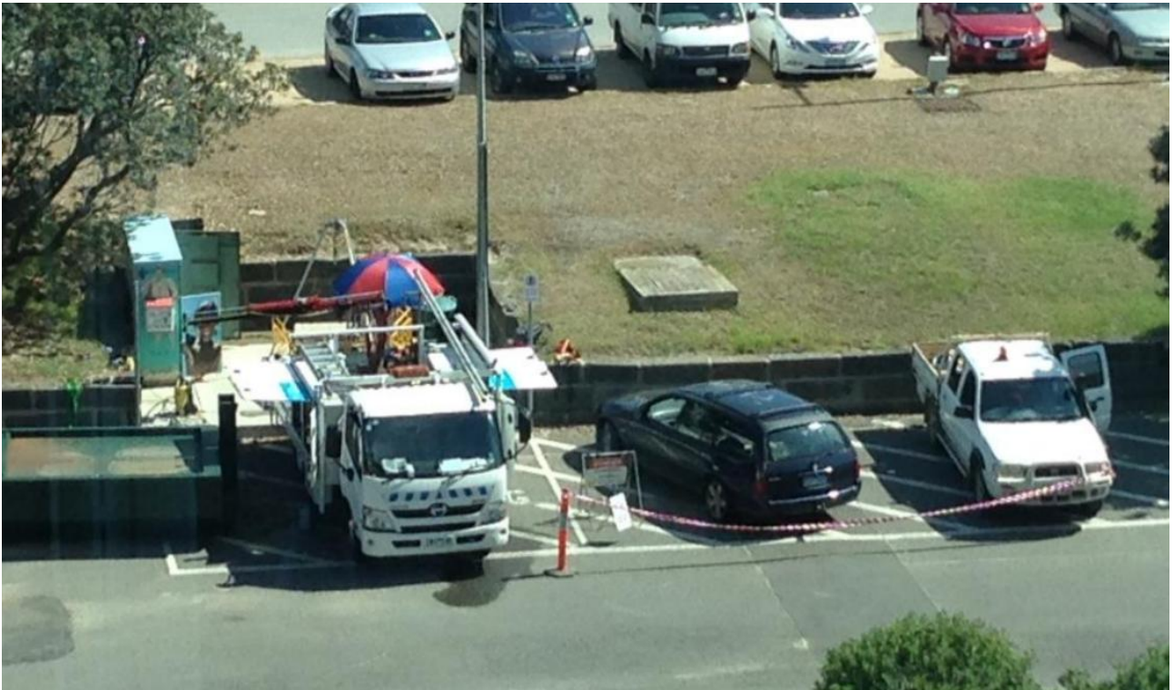
Figure 1515 - Facility set out during pump removal works
