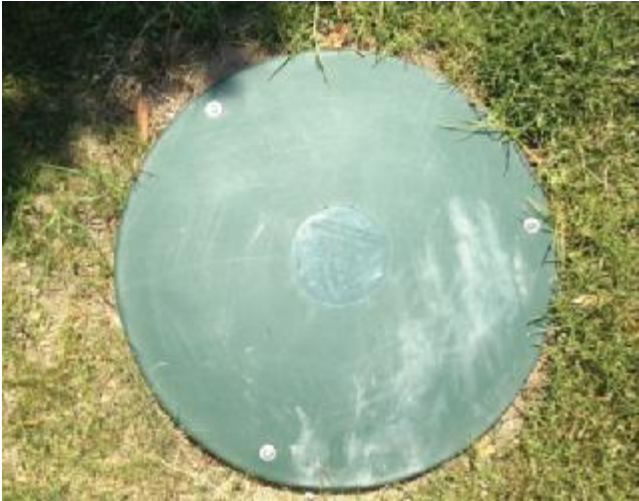
Figure 13A – Tank Unit after Installation
