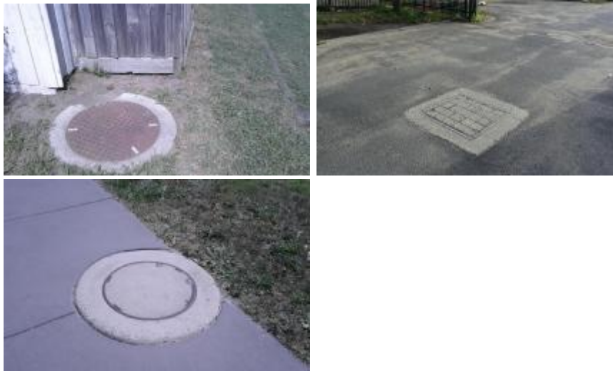
Figure 25- Maintenance holes
