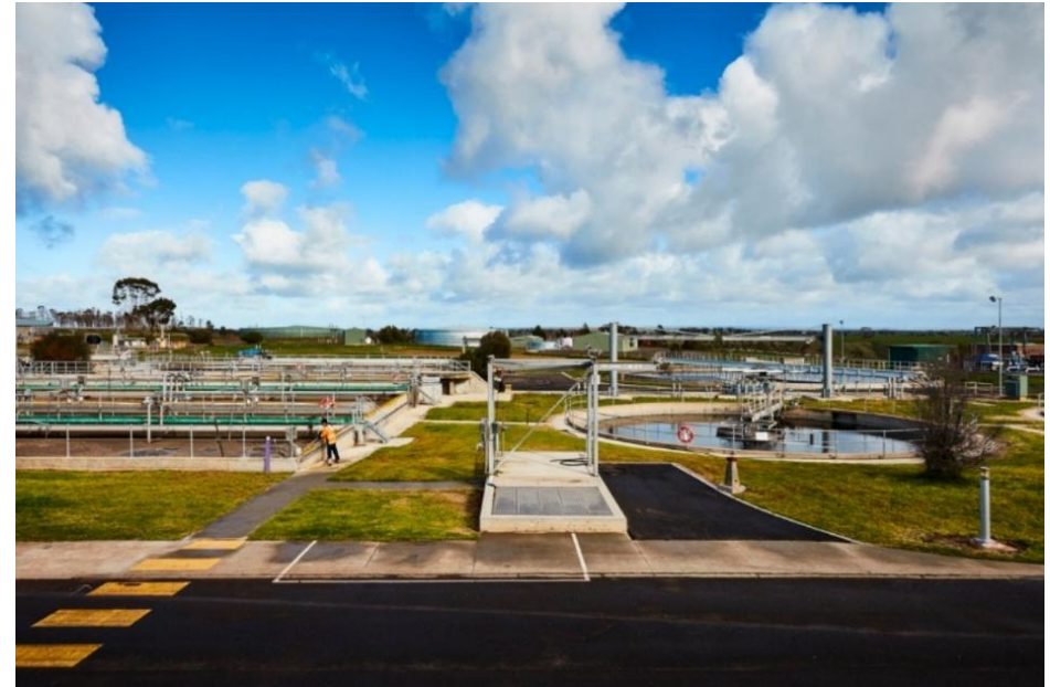
Image 5 Melton Recycled Water Plant. Credit Craig Moodie
