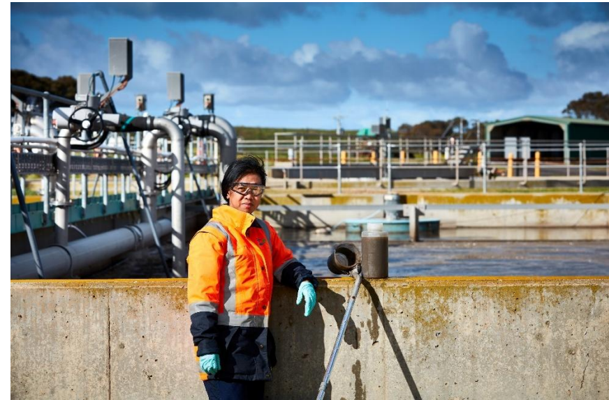
Image 8 Melton Recycled Water Plant. Credit: Craig Moodie
