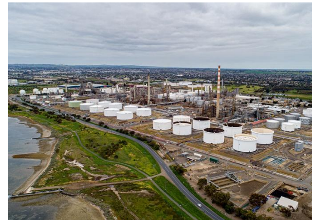
Image 1. Geelong Energy Hub. Credit Viva Energy Australia
