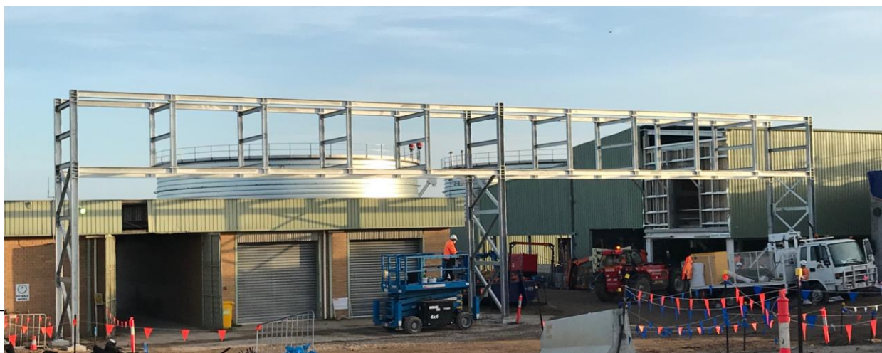
Piperack installation for Thickening Mixing Tank
