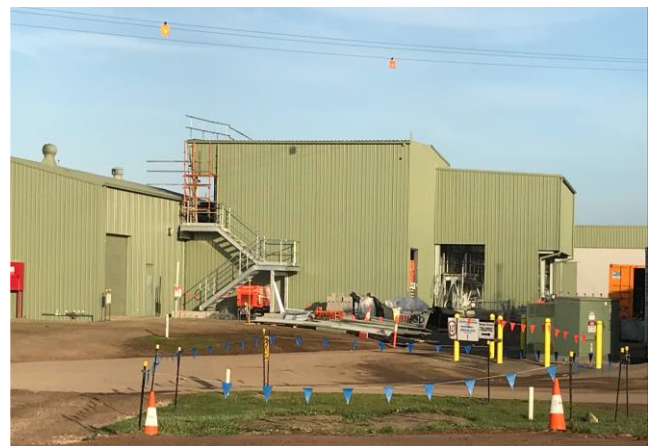
New Dewatering building
