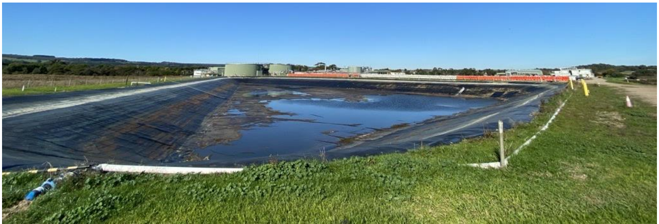
Emergency Storage Lagoon to be upgraded
