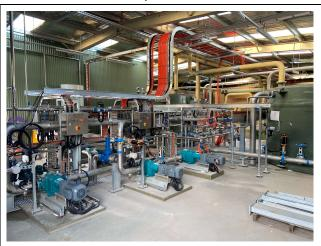
The new Tanker Receival Facility accepts waste from external septic trucks. The product is then treated and recycled on site.
