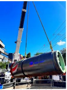
Tunnel boring machine being lowered into Worksite 2.
