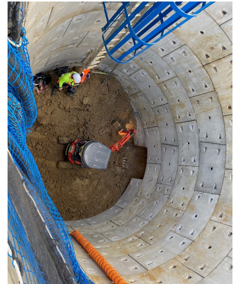
Excavating the shaft at Worksite Four.
