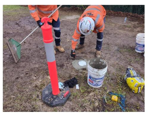
Figure 4: Well installation at BH01
