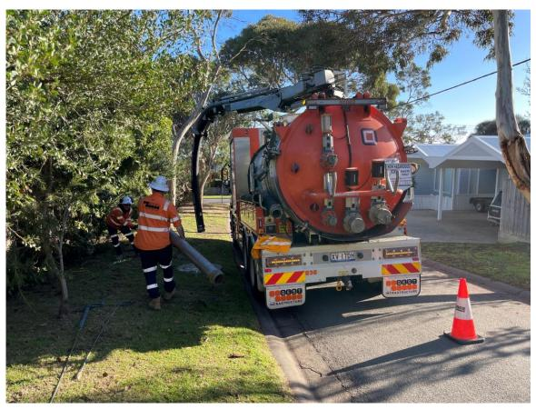
Figure 3: Non-Destructive Digging vacuum truck
