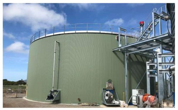
Anerobic digester with cladding
